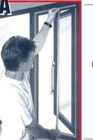
From the inside top to the(A) inside bottom of the frame -The height (A)
