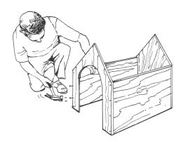
Measure the roof sections and allow an overhang at each end and at the sides. Using a saw or plane, bevel the edges of the roof to form a mitre join. Under cut the overhanging edges to help drain water off and avoid excessive moisture on the end grain. These will need to be rounded off for safety. Then glue and fasten the roof panels to the kennel. Ensure plenty of adhesive is applied to the apex joint.
