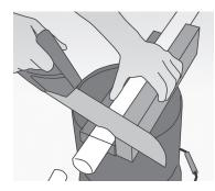
Square pipe ends fit snugly into the fittings, allowing plenty of contact area for the solvent cement to work. They also make a smoother interior surface for better water flow. A power mitre saw and other special tube cutters guarantee square cuts, but you can do the same job with a hacksaw. The illustration shows an easy-to-use guide that's made by screwing together pieces of timber.
