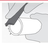
Dry fit the pipe and fitting, using a torpedo level if needed to align the fitting, and make a mark across the fitting and pipe.
