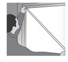
Measure the rebate (the area into which the glass will fit, including the groove in the frame) both horizontally and vertically. Double-check for squareness by measuring the diagonals, which should be equal. If your frame is not square, cut a piece of stiff cardboard to the exact size of the rebate. The glazier will use this as a template for cutting the glass to the correct size, allowing for the necessary clearance.
