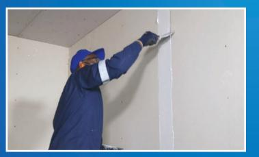
**Step 4 (a):** Reinforce the joints with RhinoTape<sup>®</sup> and apply RhinoGlide<sup>®</sup> onto the tapered edges and butt joints for a final finish.
