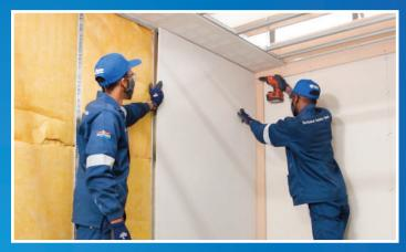
**Step 3:** Fix the RhinoBoard<sup>®</sup> 12.5 mm onto the Gypframe<sup>®</sup> UltraSTEEL<sup>®</sup> framework using Gyproc 25 mm sharp point screws.
